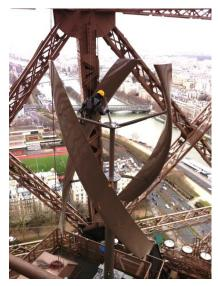
Each 7 metres high and with a 3-metre span, both wind turbines were deployed 127 metres above ground on the 2<sup>nd</sup> floor, the most suitable location for optimal windage.
