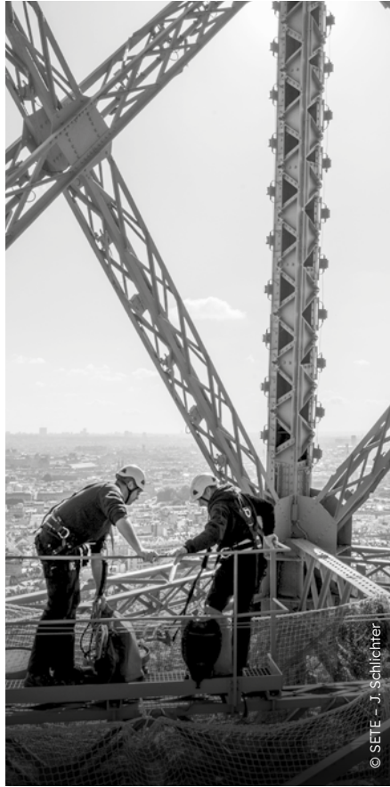
Electricians carrying out maintenance work on gold spotlights
